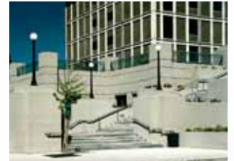
University of California Northwest Laboratory Facility Berkeley, CA
