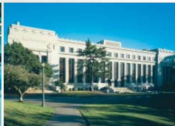
University of California, Berkeley Life Sciences; Berkeley, CA Perini renovated this 1920's building with research laboratories, museums, classrooms, and a library.
